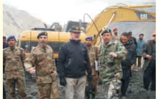
Chairman NDMA, Lt. Gen. (R) Farooq Ahmad Khan being briefed about excavation work at Hunza river blockage site
