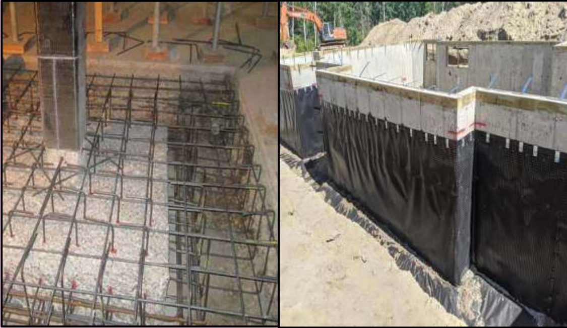
Figure 32: Reinforcement of Foundation
