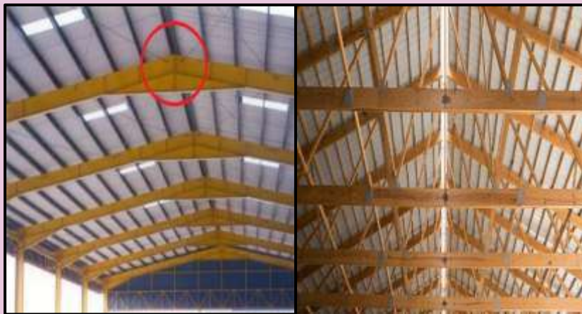
Figure 26: Roof Bracing
