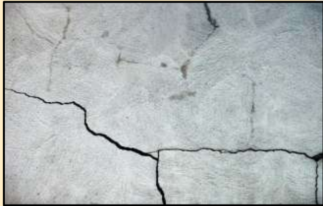
Figure 4: Cracking in a Wall
