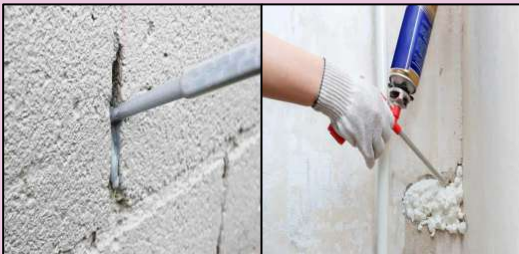
Figure 28: Grouting of Major Cracks in Walls and Columns
