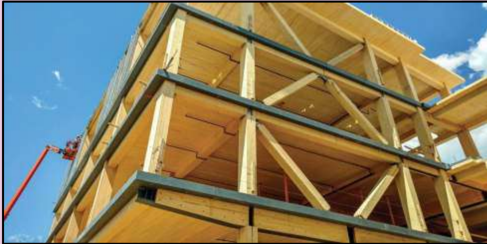
Figure 23: Timber Bracing
