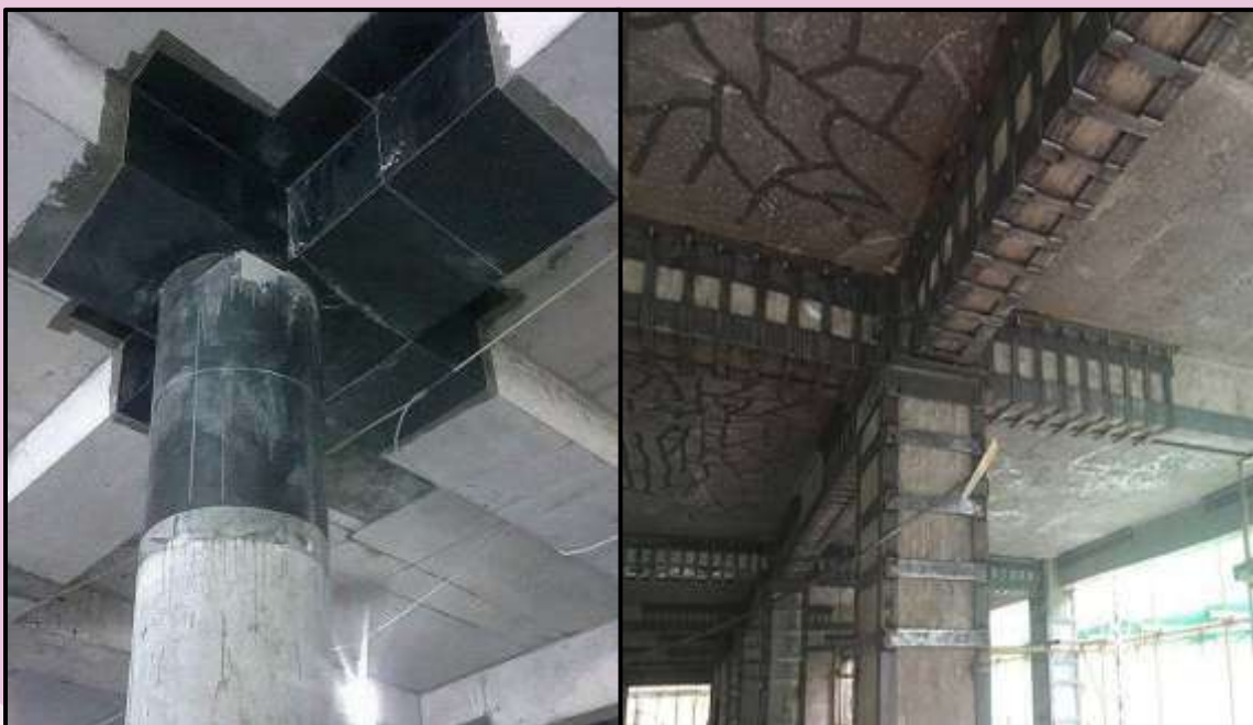
Figure 25: Beam - Column Joint Reinforcement
