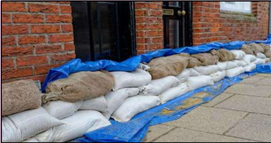
Figure 33: Sandbags Installed Around the Perimeter of House
