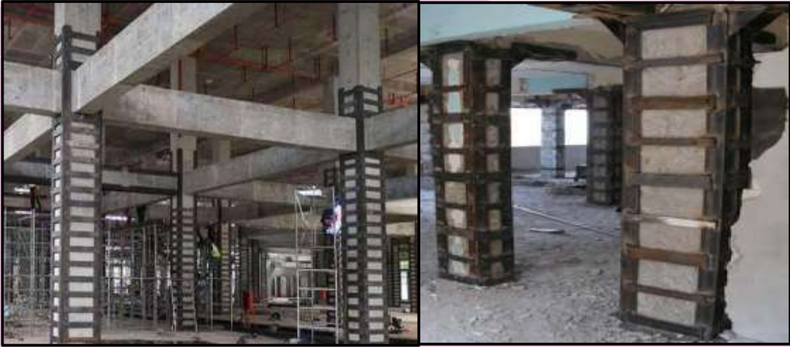
Figure 24: Column Jacketing of Existing Buildings
