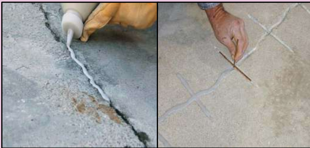
Figure 27: Cracks Filled with Grout
