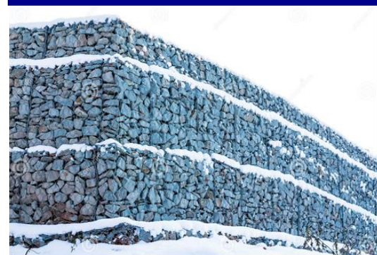
Retaining & Gabions Walls
