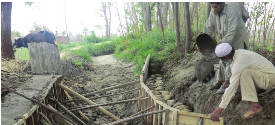
Irrigation channel mitigation measures under construction. Photo AHD
