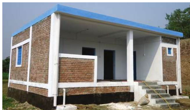
Resilient houses built to last. Photo Diakonie Katastrophenhilfe
