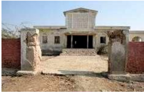
Boys School BEFORE Retrofitting
