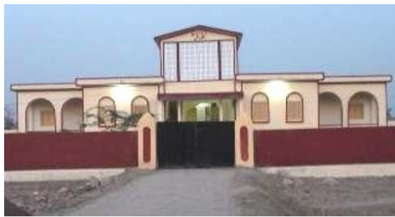
Boys School AFTER Retrofitting
