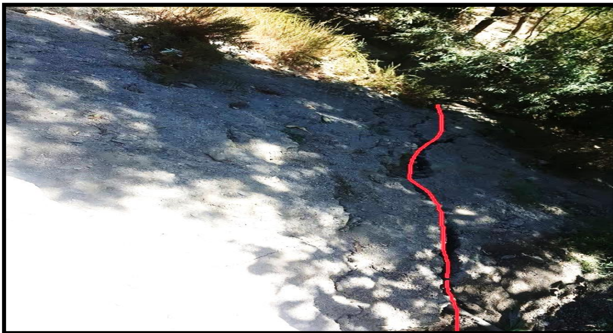
Figure 10: Deep Cracks touching bedrocks
