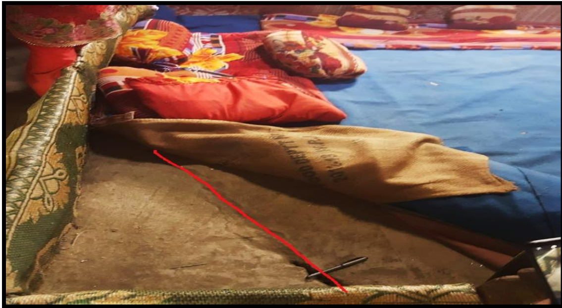
Figure 13: Cracks developed within the Houses
