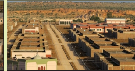
View of houses constructed at Thatta, Sindh
