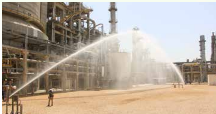
Fire water curtain formation by emergency team
