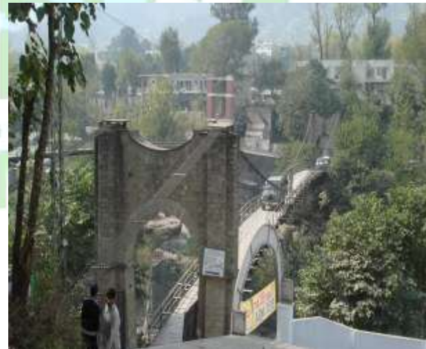
Fig:7.3 Suspension Bridge selected for retrofitting
