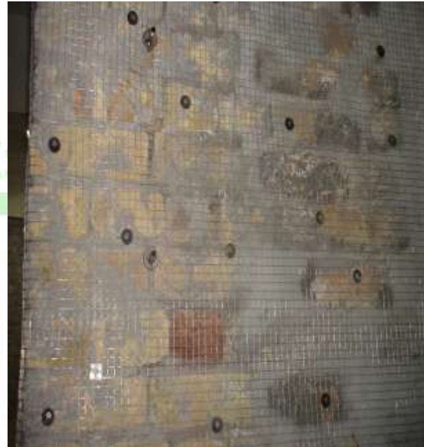
Fig:7.2 Retrofitted Wall of Jinnah Dental Hospital
