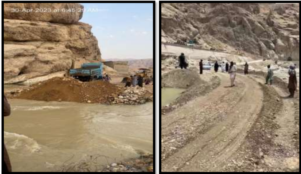
Restoration work on Pinjra bridge, in District Kohlu
