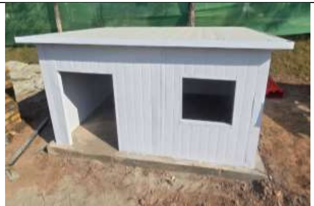
Pre-Fabricated House Structure
