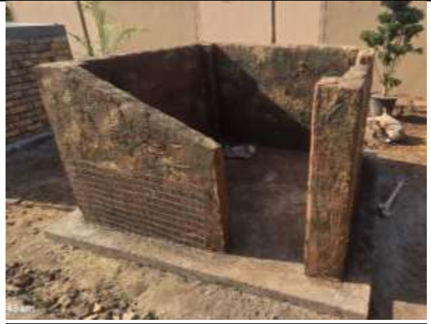
Reinforced Adobe Structure
